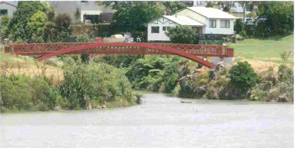
Mudlarks bridge across Owens Rd Creek.
