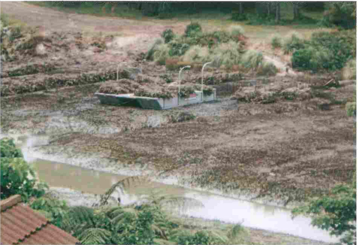
Tamakae Estuary, work in progress.
